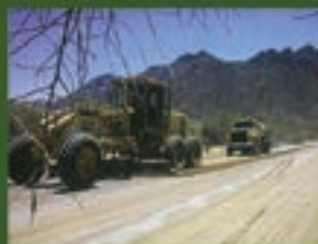
Sub-Base Stabilization
